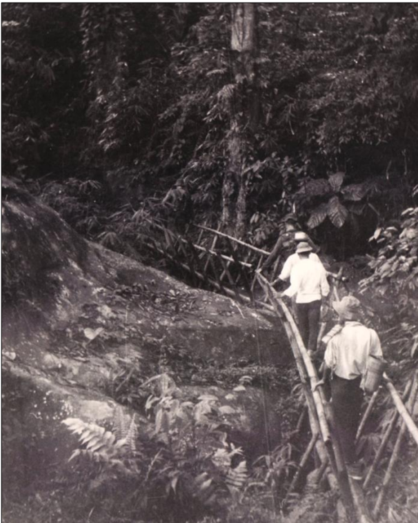
A patrol with Iban Trackers crossing a river on a traditional V-shaped bamboo bridge, called 'Tiboyant' in Bidayuh. The modern Darul Hana Bridge in Kuching was inspired by this traditional Bidayuh bamboo bridge design.
